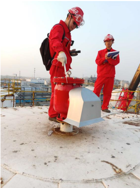
Picture 3: The customer tested leakage of PROTEGO® valves
