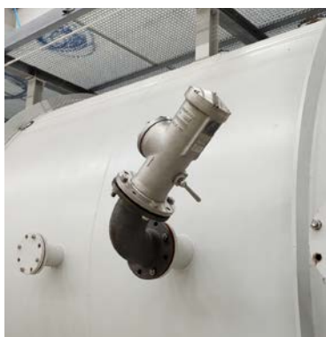
Angled installation of PROTEGO® DE/S
