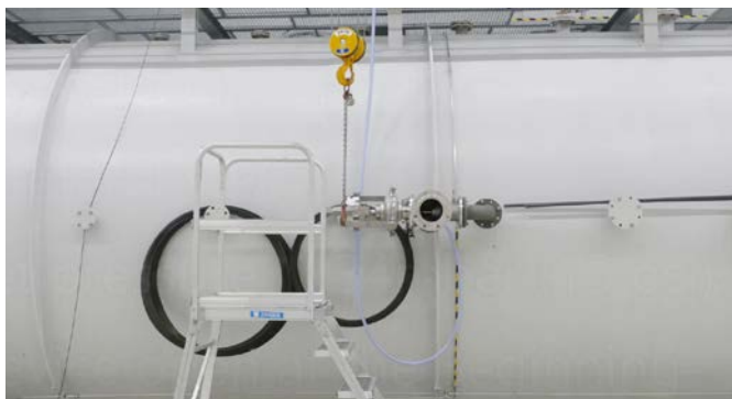
Testing the functionality of Pilot Valve when angled by 90 degrees
