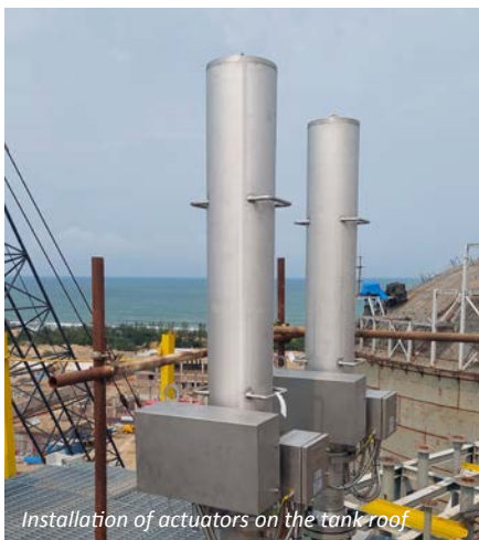
ITV-S valves in the tank
